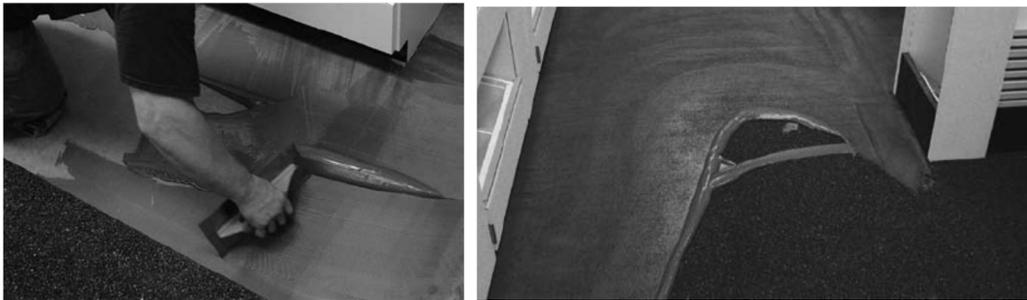
**VII. Field Lamination – Step 3 – Preparation of the 3.2mm ECOfit Finished floor surface**
