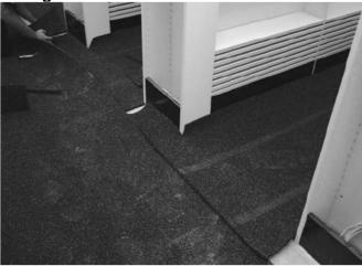
B. After all above procedures are performed, begin application of selected adhesive. Apply adhesive to the substrate using recommended 1/16" square notch trowel. Take care not to spread more adhesive than can be covered by flooring and rolled within 30 minutes. The open time of the adhesive is 30–40 minutes at 70° F and 50% relative humidity.
